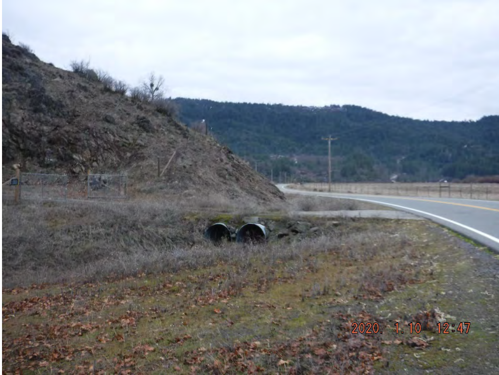
Photo #5: Two 48" CMP culverts under the access road and to adjacent Ruth Zenia Road
