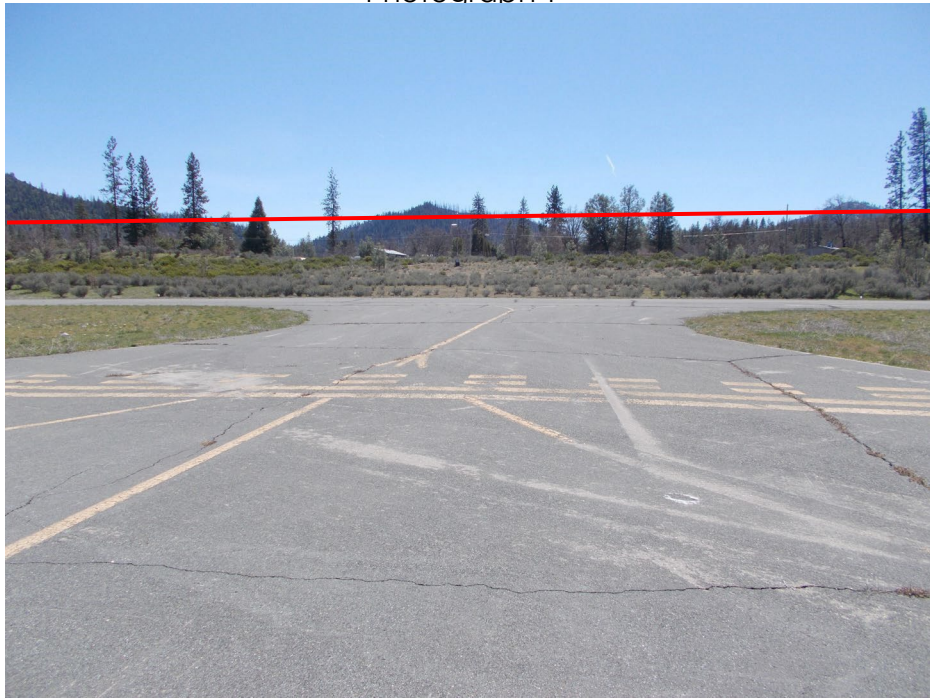
Multiple trees and power poles penetrating the south FAR Part 77, 7:1 Transitional Surface
