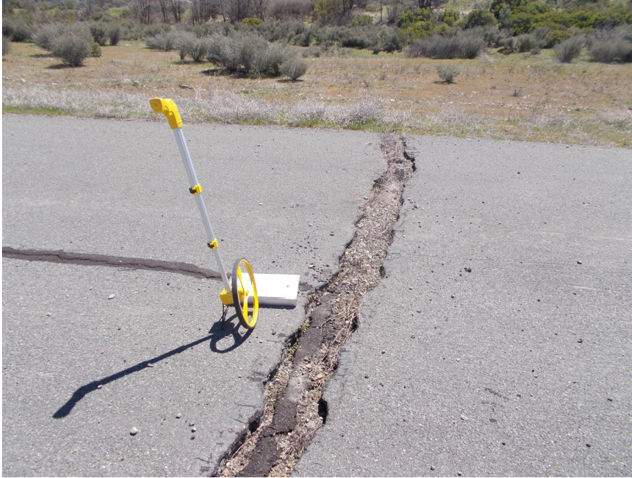
Large cracks on runway and taxiways.
